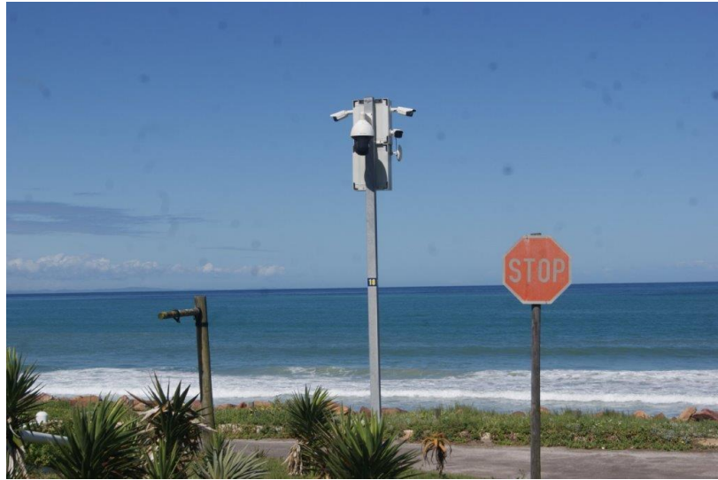
Figure 2 Typical CCTV pole
