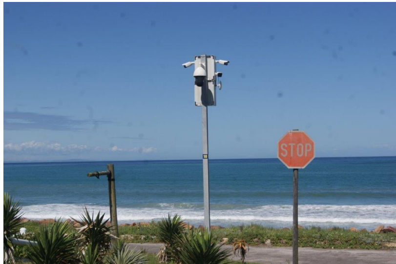
Figure 2 Typical CCTV pole
